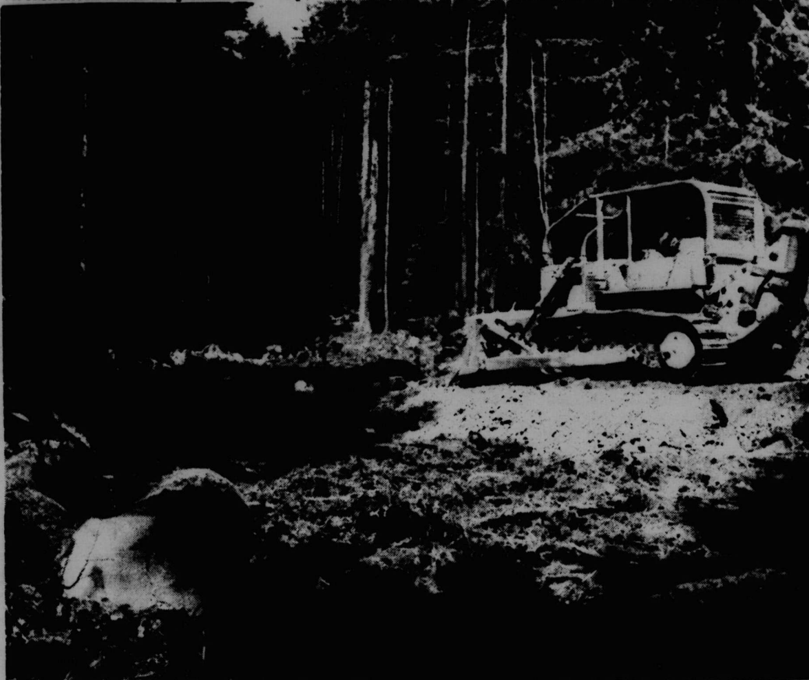
A Pacific Lumber Co. bulldozer starts work on a road for the Freshwater forest. This is the first step in the logging
