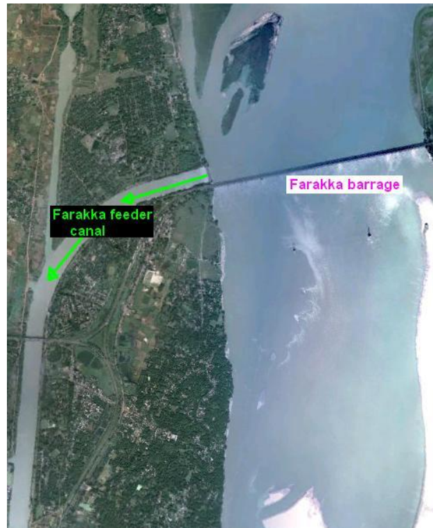
Figure 7: Farakka Barrage and its feeder channel (Foundation, Concrete, and Earthquake Engineering)
