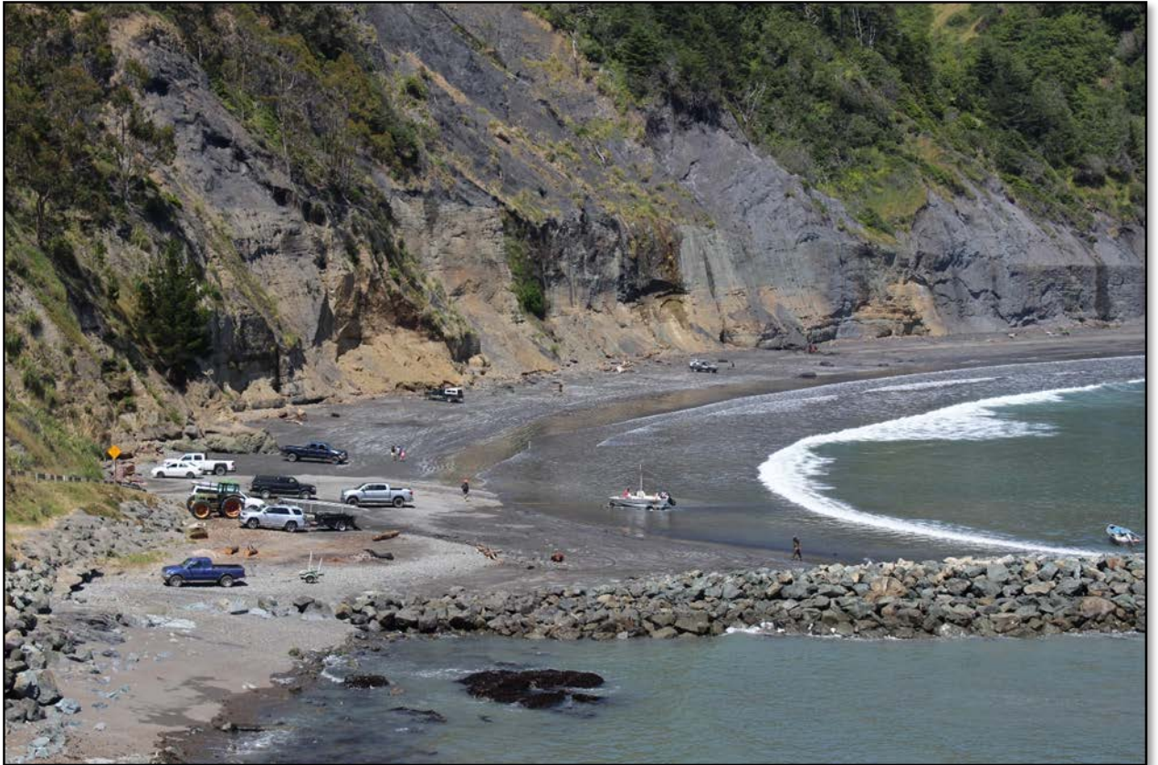
Figure 9. Boat launching facility at Shelter Cove includes road from the bluff down to the beach, boat ramp, the jetty, and the ocean. Note the tractors, trailers, and trucks used to get vessels in and out of the water (Photo: Dumouchel, 2017).
