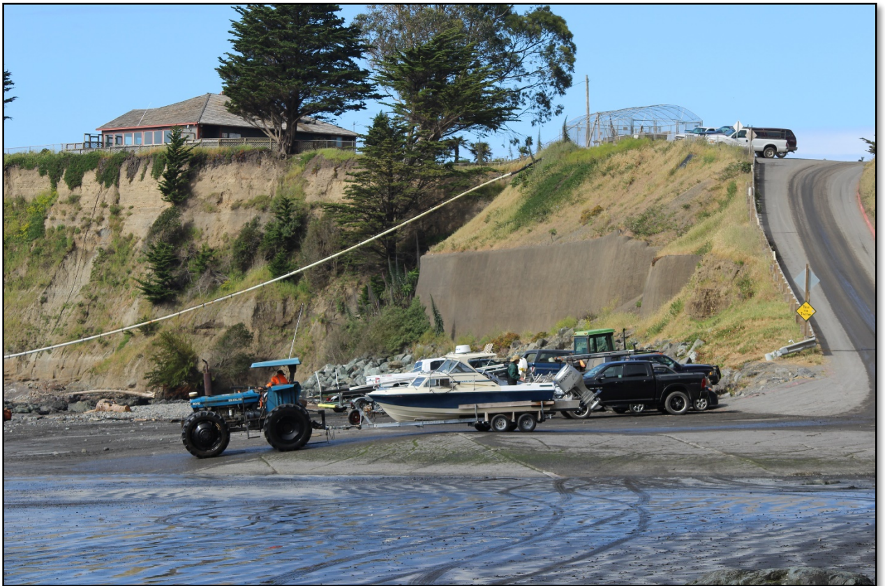
Figure 11. Shelter Cove's infrastructure includes the fish cleaning station (above bluff) and the retaining wall, "storm drain", boat ramp cement skirt, and the jetty. (Photo: Dumouchel, 2017).
