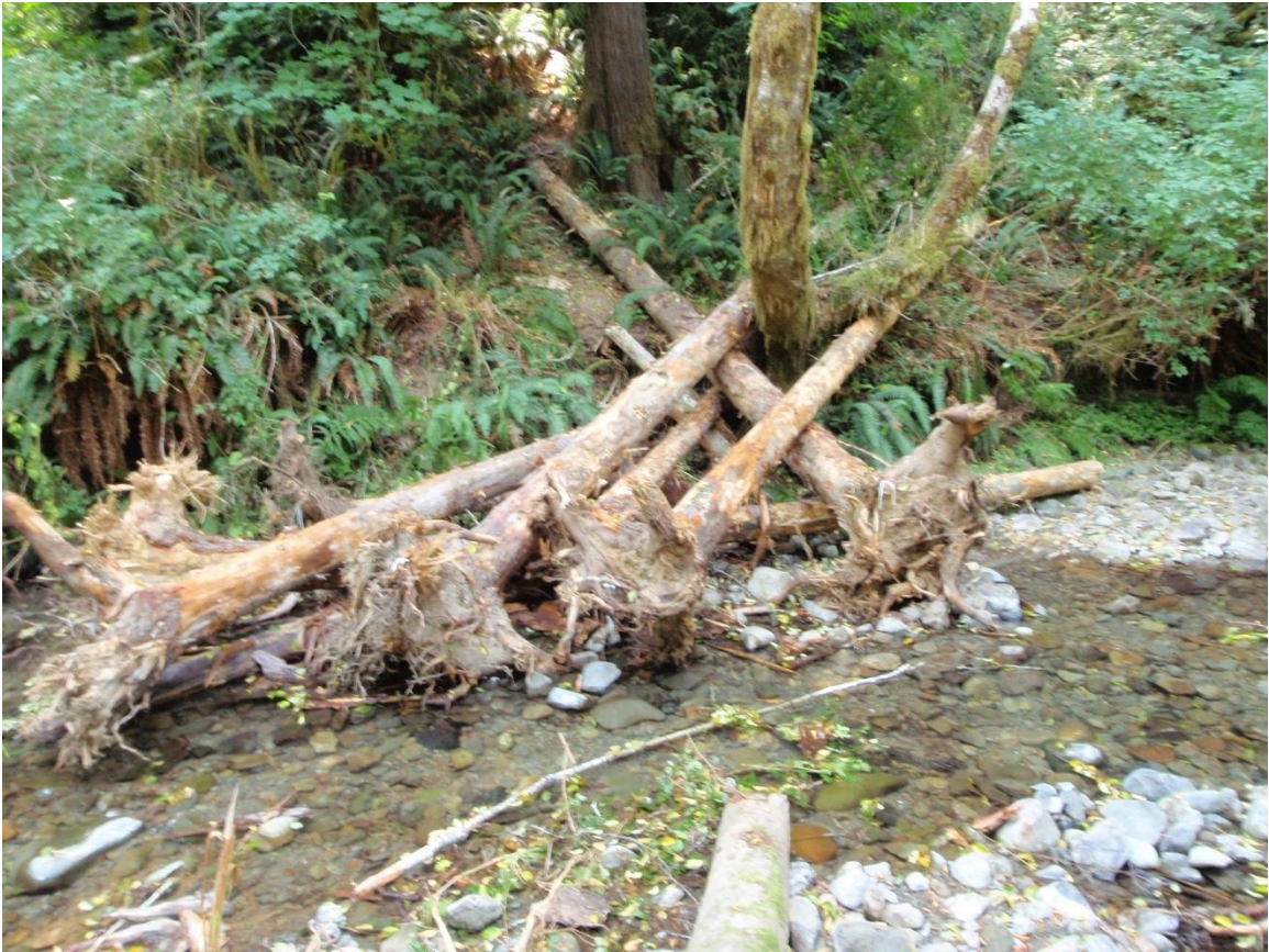
Figure 3. Complex log jam structure installed in 2008 by National and California State Parks in East Fork Mill Creek, Del Norte County, California (Flannery 2011).
