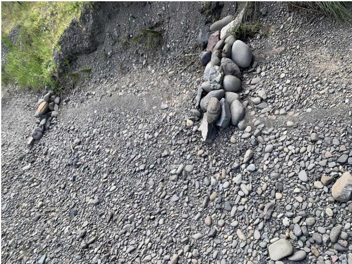
Figure 7: Fine sediment behind rock weirs at the toe of the eroded slope (Sebastian Castillo)
