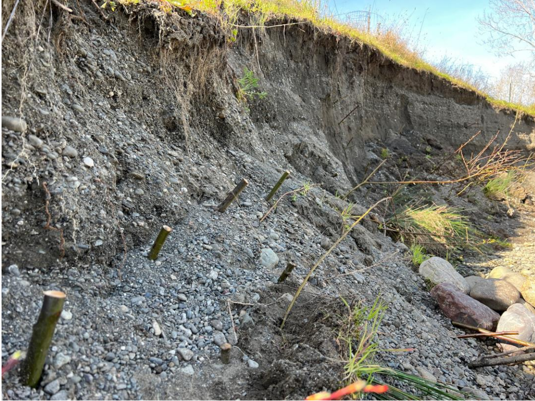
Figure 5: Salix spp. and Juncus spp. transplant on the eroded bank (Daniel Price).
