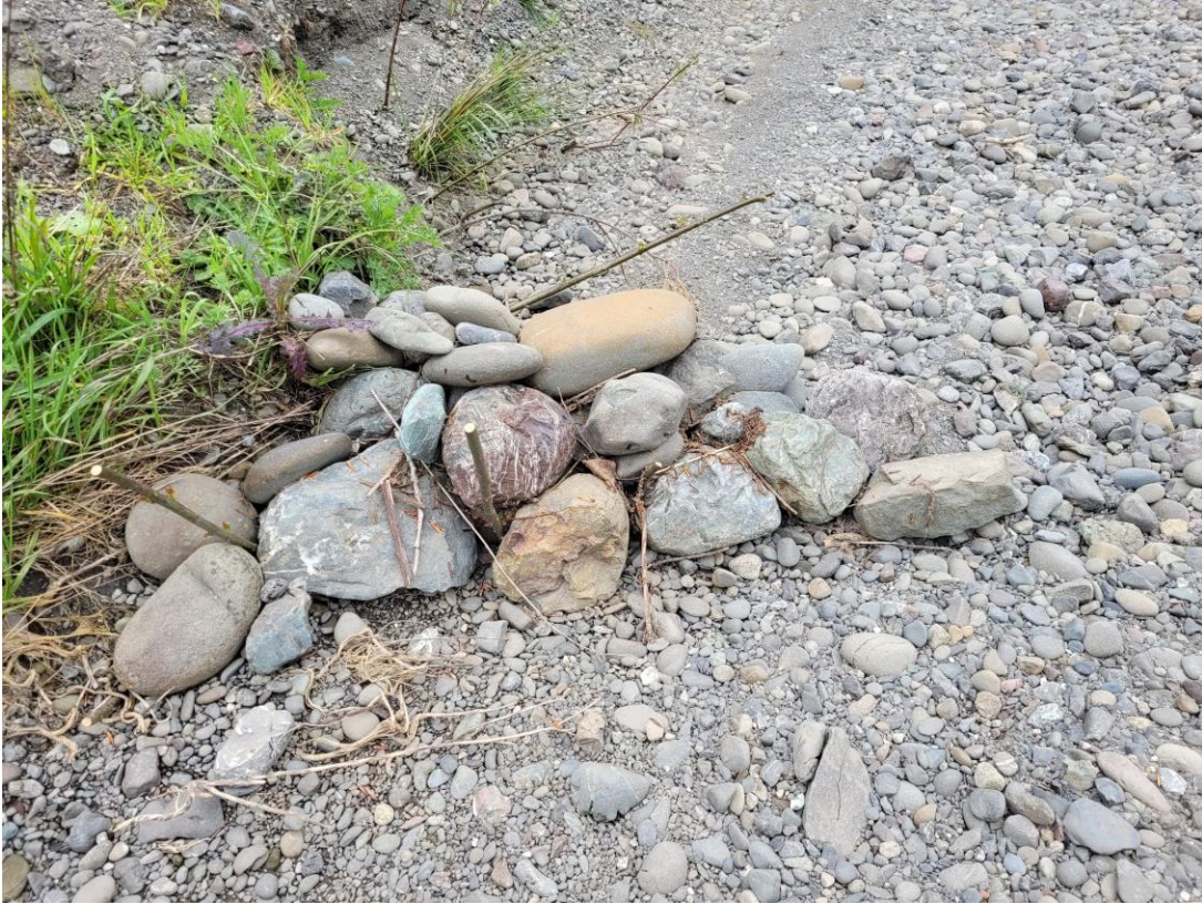
Figure 4: Constructed Rock weirs (Daniel Price).
