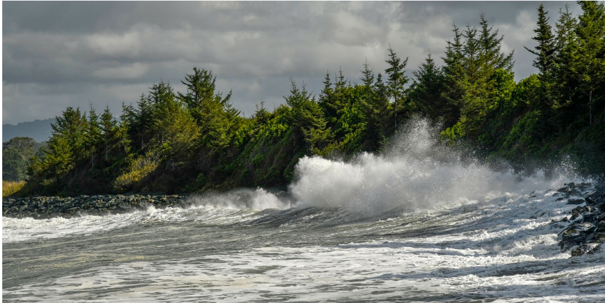
King tide waves overtopping the sea wall at Durouk Higuchguk where nuclear fuel is being stored.
