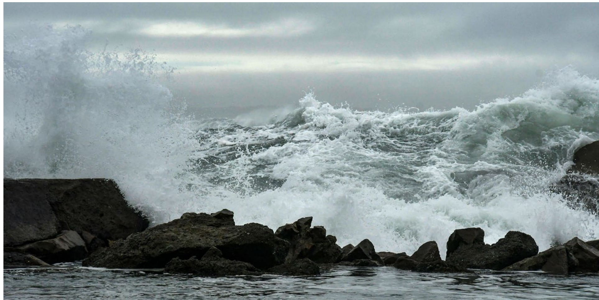
Stormwater waves on the North Jetty.
