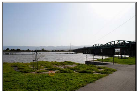
The Eureka Slough and the Highway 101 Bridge, taken from behind Target in Eureka. Photo by Carrie Carter-Griffin (4/22/10)
