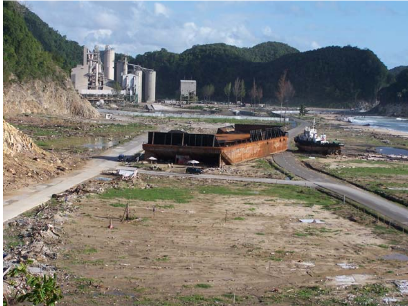
LaFarge cement plant is in the background. Tsunami wave run up at this location was measured to be 38.9 meters (~128 feet) (SN 5/2005)
