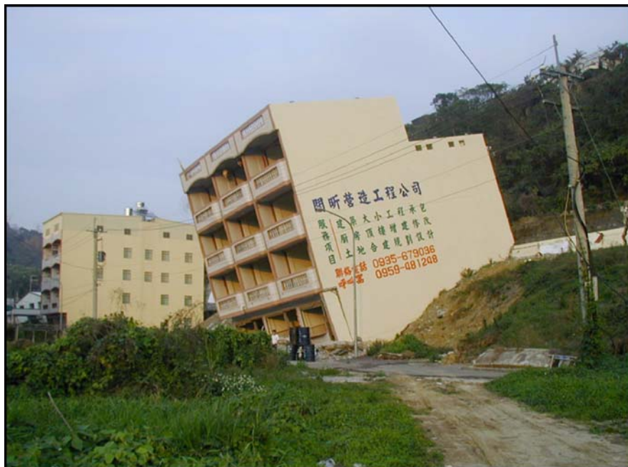
The rigid reinforced concrete building is tilted on the forelimb at tip of fault-bend fold (WDP 2000)
