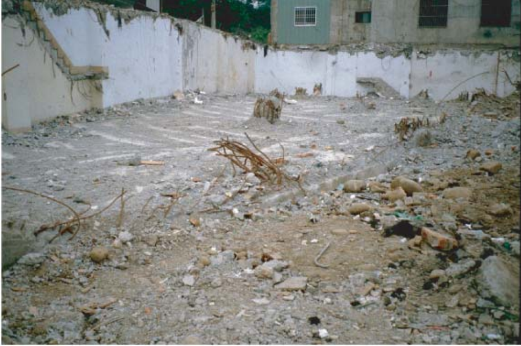
A) Fault bend fold appears as flexure on the floor of a building destroyed by surface faulting during the 1999 Chi-Chi earthquake.
