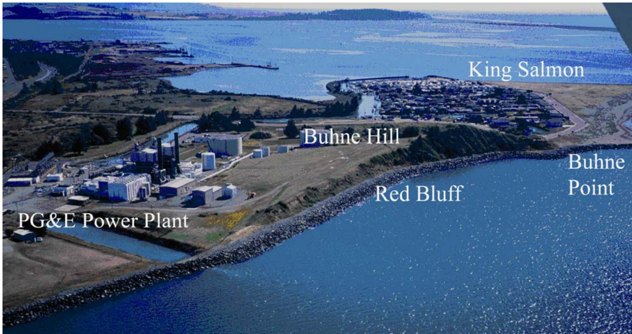
View to southwest; the ISFSI site is below the 'e' in Buhne Hill
