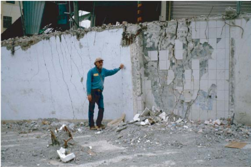
B) Shears and fractures in wall over the fault bend fold shown above in Photo 8-3A.
