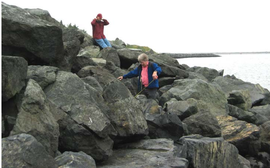
Photo 5-6 Twenty degree slope of riprap in berm in front of Red Bluff
