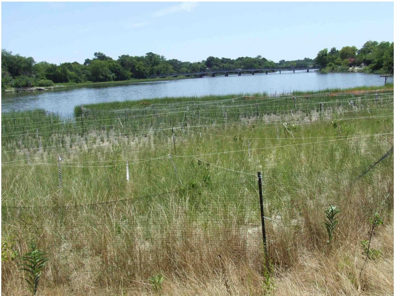
Figure 12: Photo by K. Duhring. Here a recently planted marsh is being protected from grazers to ensure a successful take of the vegetation. 9
