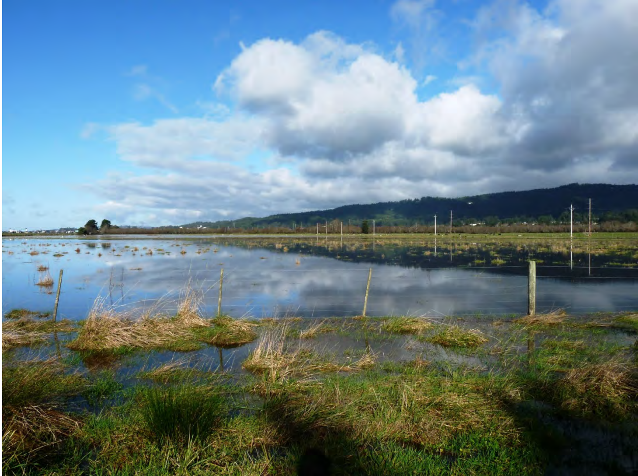
Figure 24. Highway 101 traverses several tributaries and streams to Arcata Bay that convey stormwater runoff and can flood land to the east of Highway 101.
