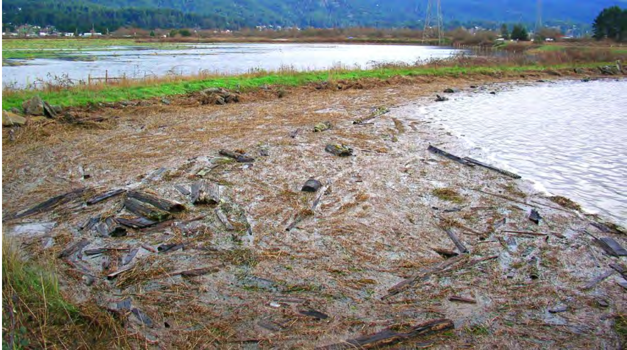
Figure 1. New Year's Eve 2005 king tide with dikes filled to overtopping in Arcata.
