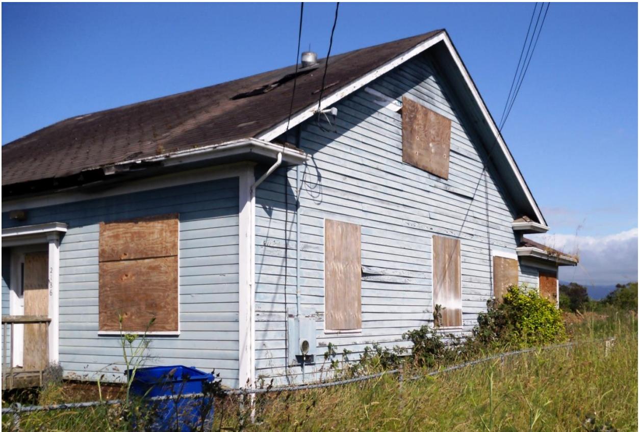
South elevation showing recessed entry, cornice returns, southeast corner. Photo May 2015.
