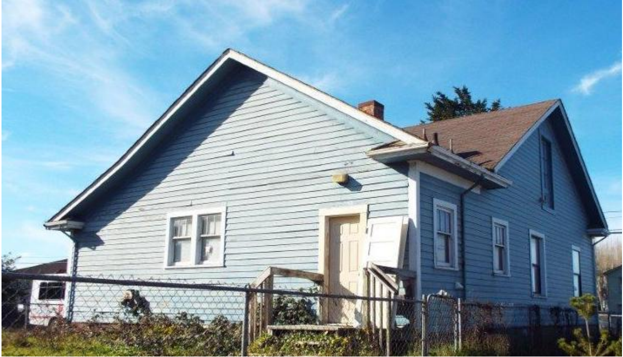
East elevation showing windows with upper divisions and modern door Photo Jamie Roscoe Feb. 2015.
