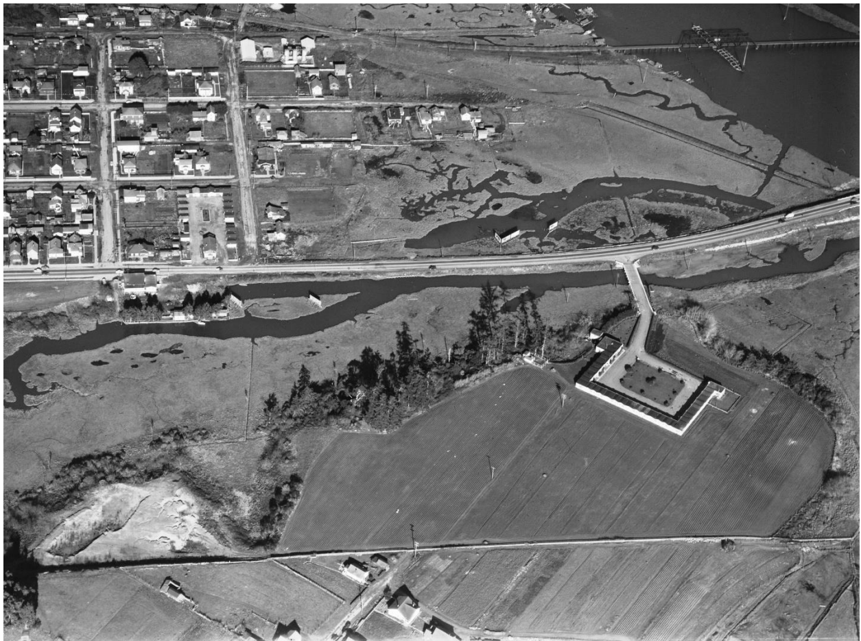
Hotel Court on flat across highway slough. Tydd Street house at very bottom of photo. Shuster Photo, 2001.01.0058. HSU coll. Online. Photo 27 Dec. 1946.
