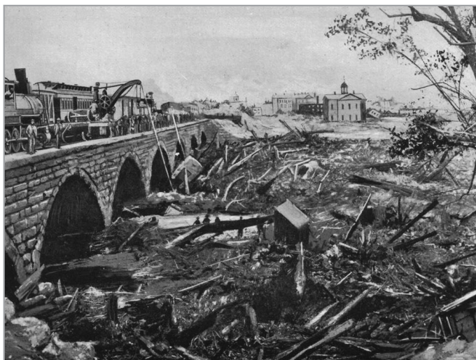
Debris and devastation washed against Stone Bridge in the wake of the Johnstown Flood. (Public Domain.)
