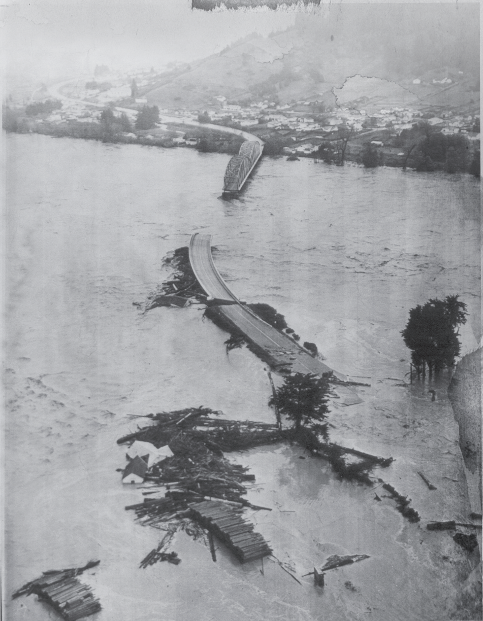
(EK2) RIO DELL, CALIF., Dec 23---Bridge Out--- Highway 101 bridge is out at the town of Rio Dell 28 miles south of Eureka, as the Eel River takes a toll of homes, farms and roads and bridges
